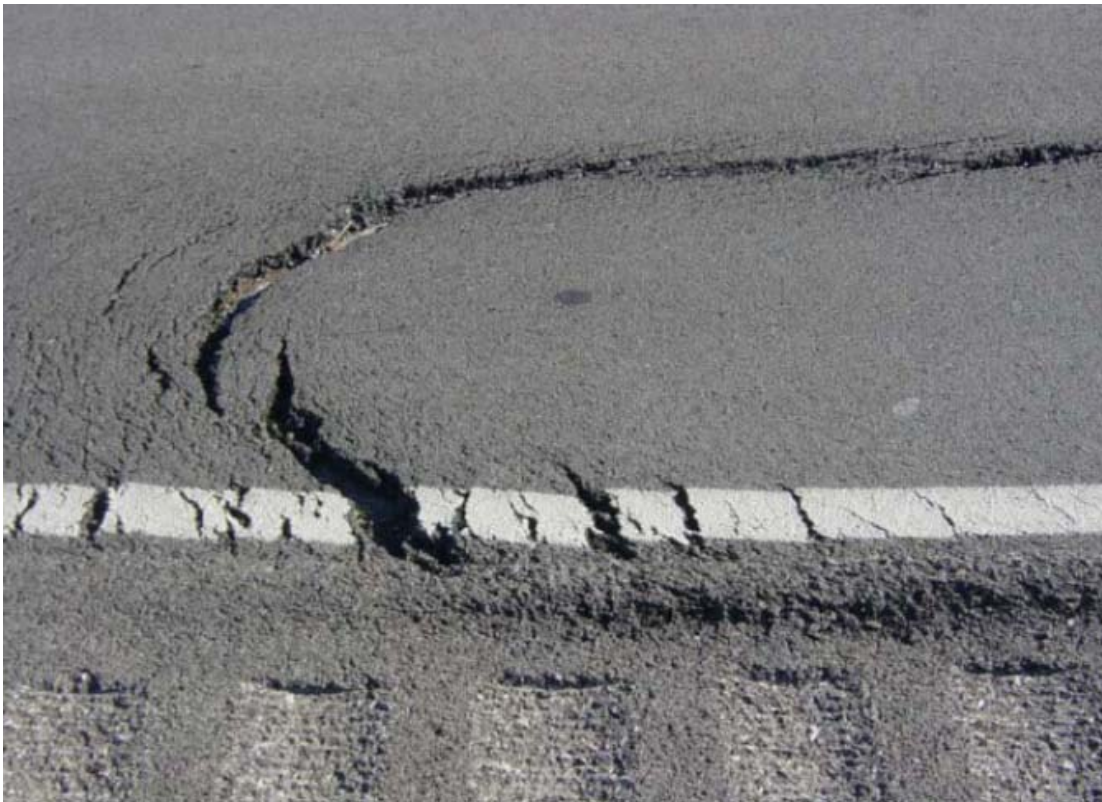
FIGURE 1 Slippage Cracks (14)
