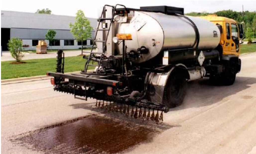
FIGURE 2 Tack Coat Distributor (3)
